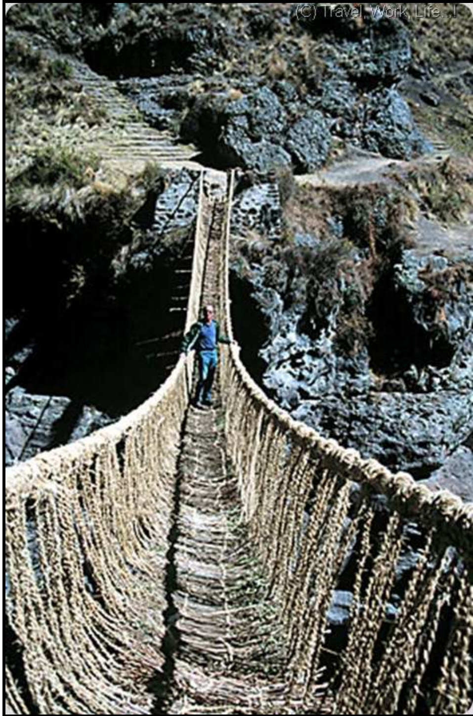
Replica of an Incan rope bridge built in the Apurimac region, south of Cuzco.
